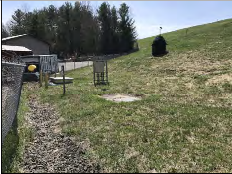
SCENE: View facing southeast of the northern toe of the landfill cap and the leachate management tank. DATE: May 2, 2018
