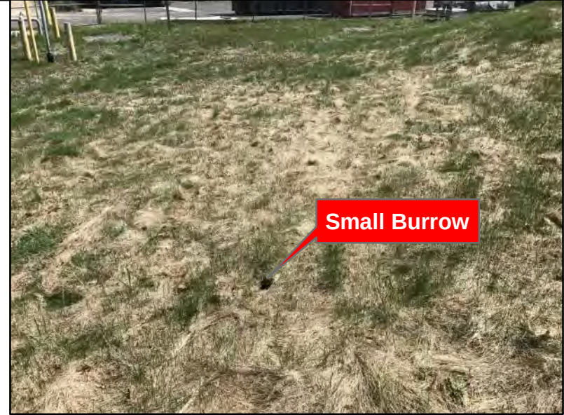
SCENE: View facing east of a small animal burrow in the landfill vegetated layer. DATE: May 2, 2018
