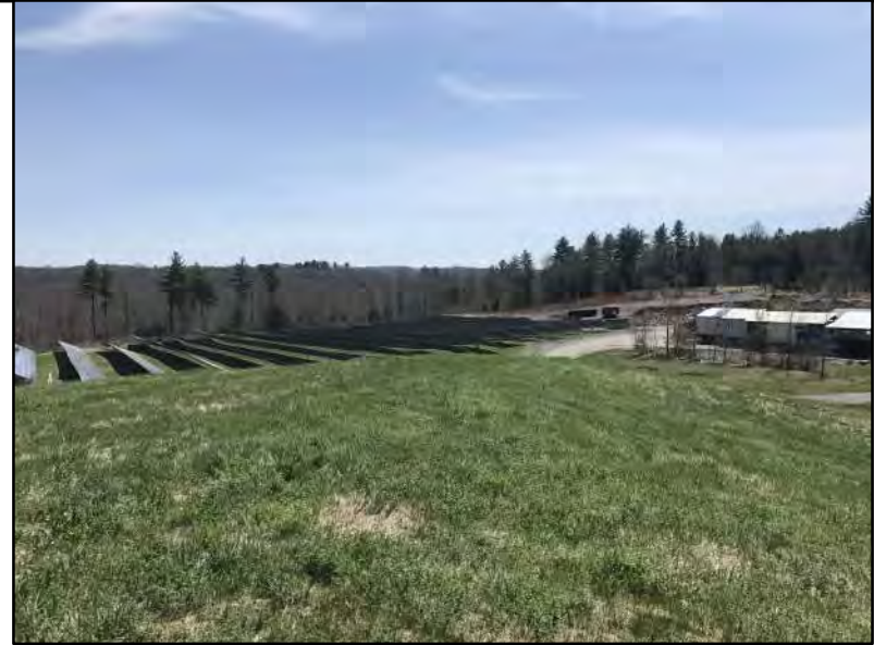
SCENE: View facing southeast the solar array and bulky waste management area.. DATE: May 2, 2018
