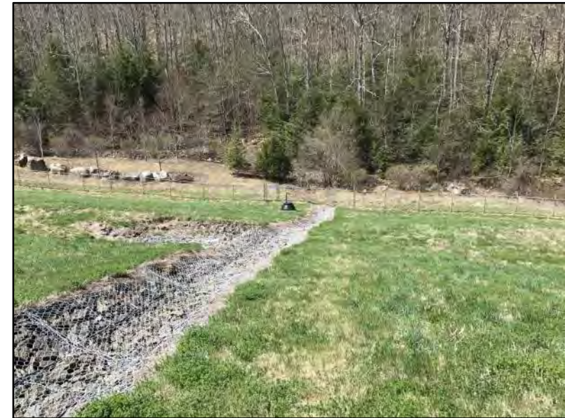
SCENE: View facing west of the western downchute and manhole MH-1. Water was noted flowing in the downchute. DATE: May 2, 2018
