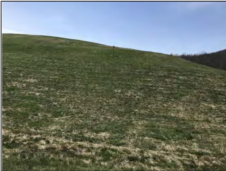
SCENE: View facing south of the north-facing landfill slope. The remaining landfill slopes were in similar condition. DATE: May 2, 2018
